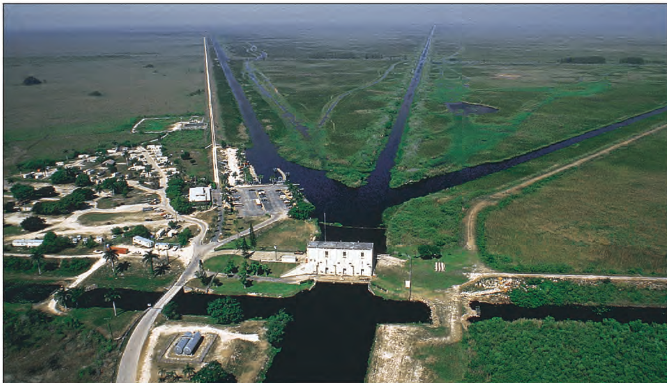
Photo 1. S-9, a retrofitted pumpstation and its environs
