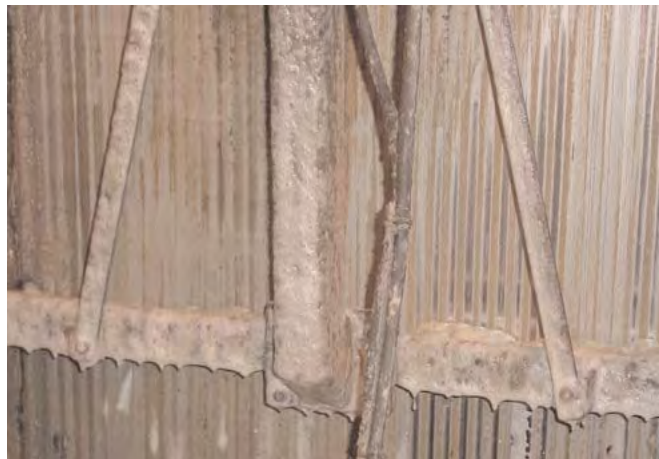
Bar Screen with Rake
