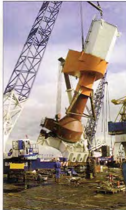
Loadout of the Libyan FPSO turret at Burntisland.
