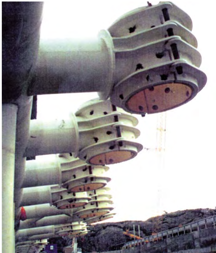
Bearing support structure
